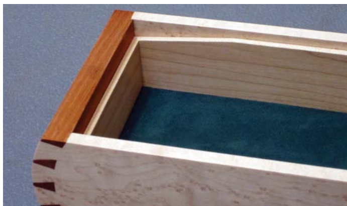
The angled lining in place
