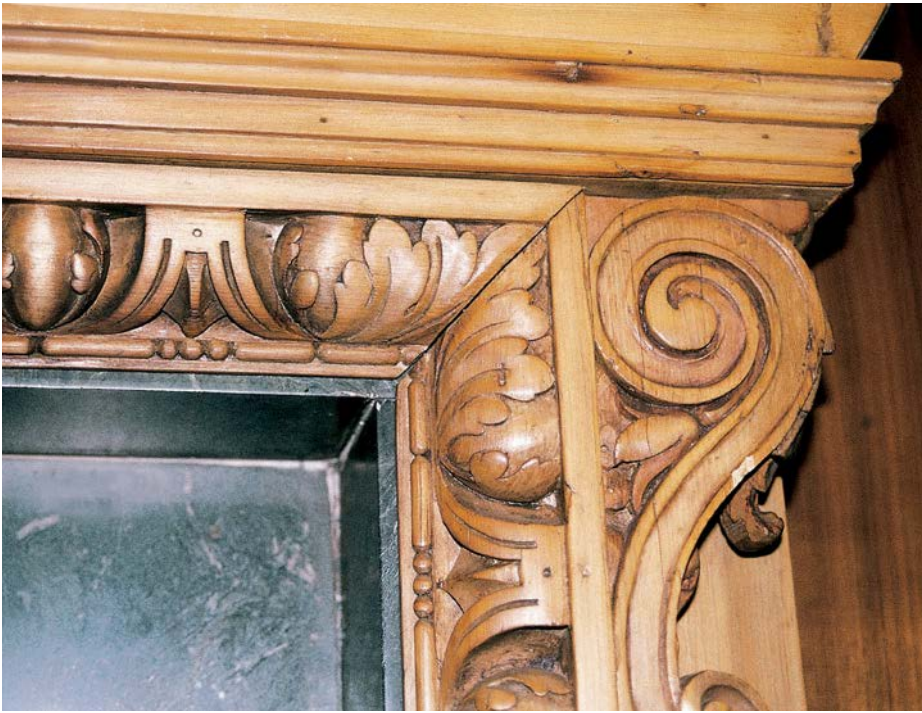
Fig 7: Egg and dart moulding, showing the use of leaves to mask the mitre joint
