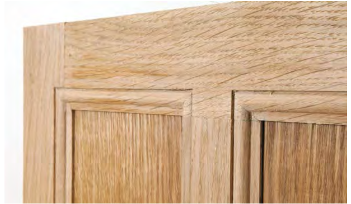
Not the most elegant way of getting a moulding round a corner
