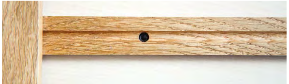
Machine screws are located in the slides to act as either a stop or a hook
