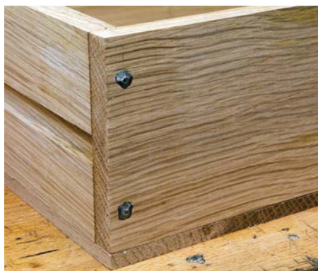
The back is just a butt joint and cut nails
