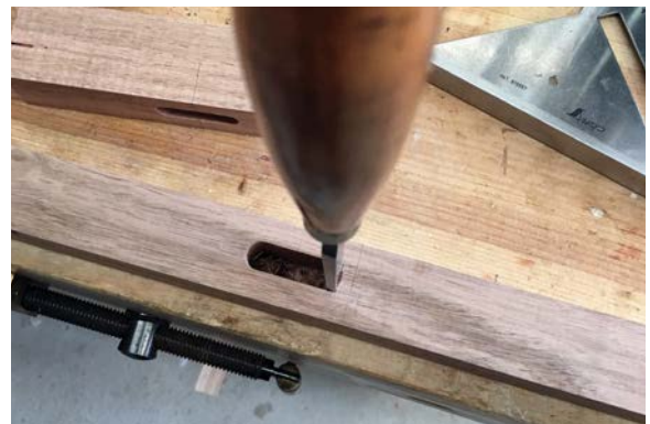
Squaring up the mortise
