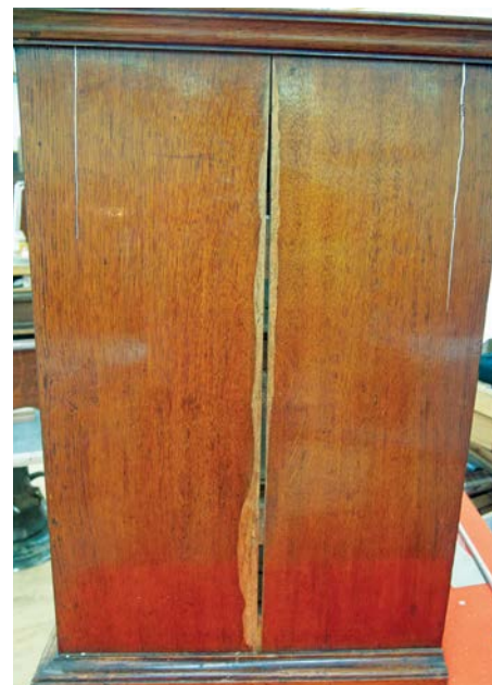
The side of the chest after removing the previous oak sliver from the big centre split
