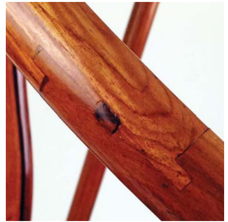
A peg forces the interlocking parts together
