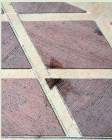
Carry out any repairs with offcuts of veneer
