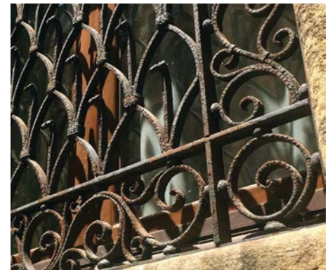
Ironwork detail seen in Brindisi
