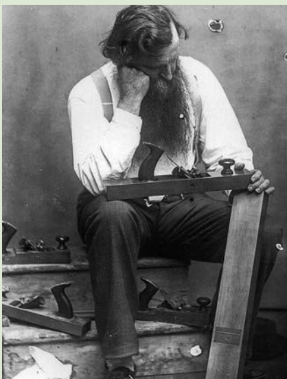
John Porcius Gage surrounded by Gage Tool Co planes. The bottom of the iron blade box is clearly visible in the sole of the long plane in the foreground
