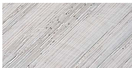
Pay attention to air bubbles and loose dust in the open grain of the wood
