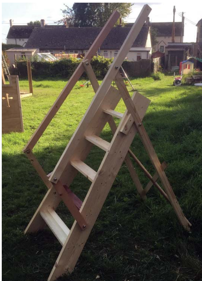
Mock-up of full-size steps in softwood screwed together and left as square edge for speed
