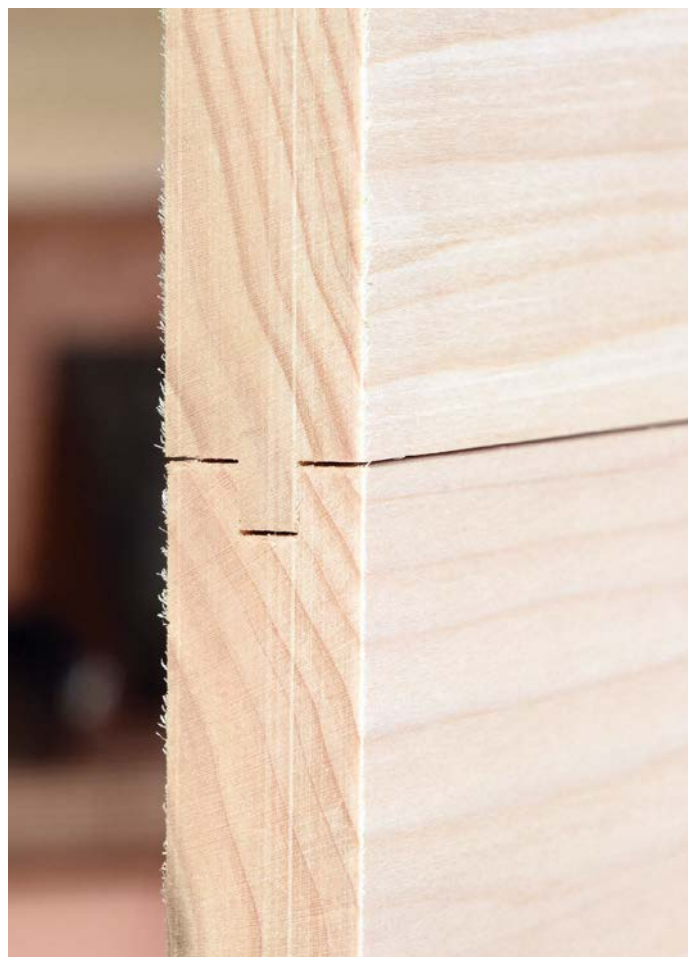
As a glue joint it offers little strength but great alignment
