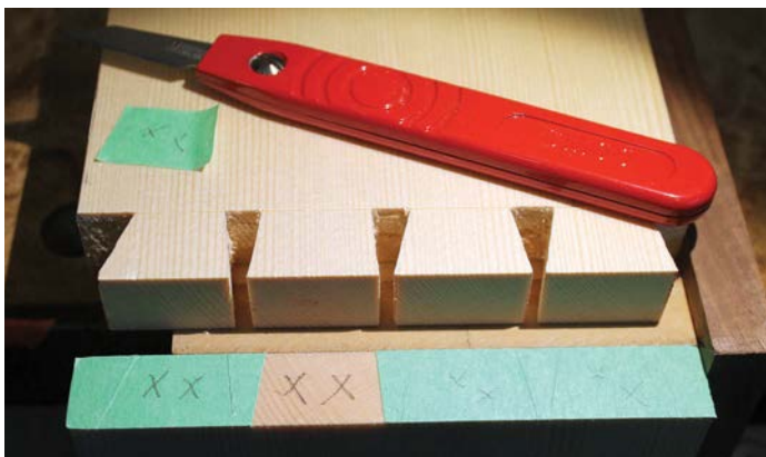
Mark the waste on the tape as soon as you knife the lines to prevent any peeling mistake
