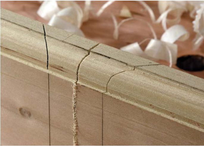
Check that adjoining corners have the same profile
