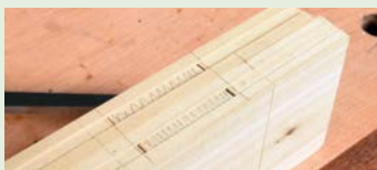
Create a groove to set the mortise in place and guide the chisel's first cuts
