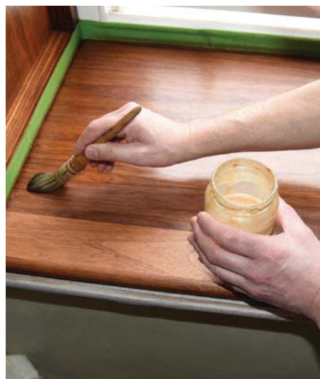
Sealing oil stain in place with shellac sanding sealer
