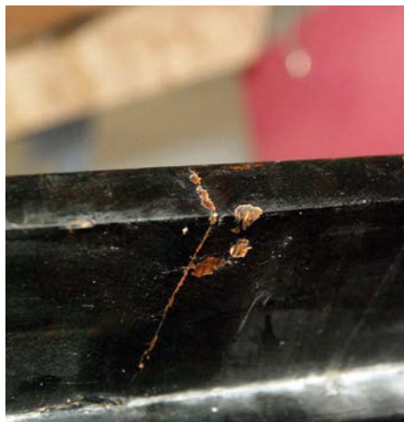
Holes drilled to enable the groundwork to be realigned
