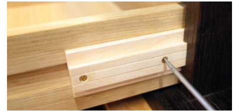
The drawer is installed by screwing in the fillets
