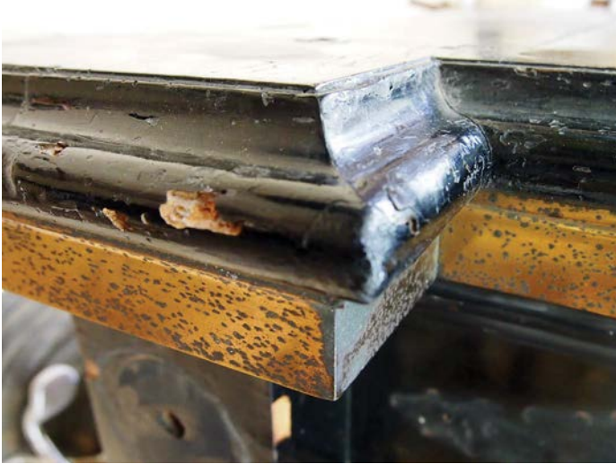
Areas rebuilt with shellac filler and sawdust with animal glue
