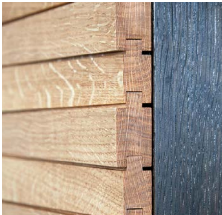
The door is made up of 10 individually tapered staves, which are threaded onto concealed batons
