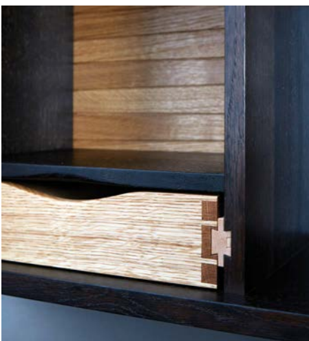
Full extension drawer runners run in dovetail housings in the drawer side and carcass
