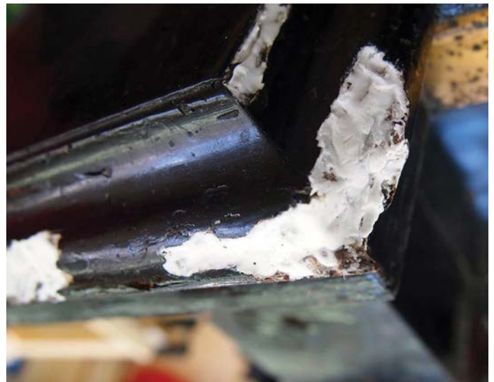
A thick paste was added as the second part of the barrier layer
