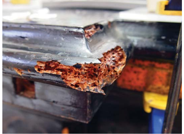
The previous fillers were removed
