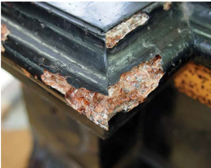
The damaged wood was consolidated and Japanese tissue was applied
