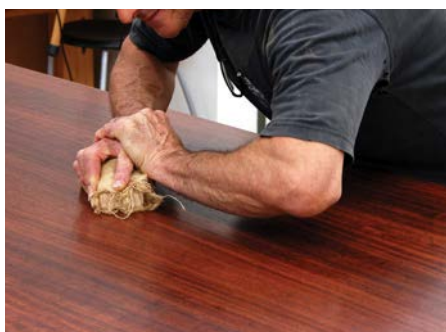
You need to rub hard and vigorously along the grain
