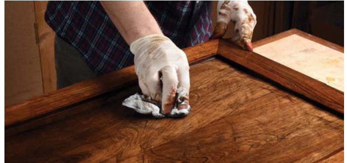
Work the stipple into the corners and edges and leave to dry before setting with shellac
