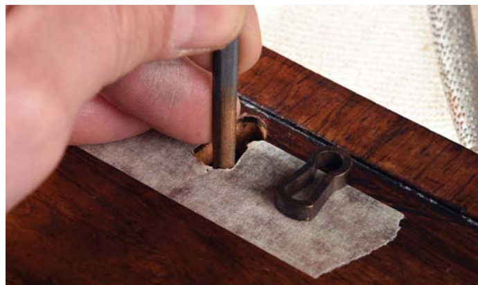
Use files or rasps to expand the hole
