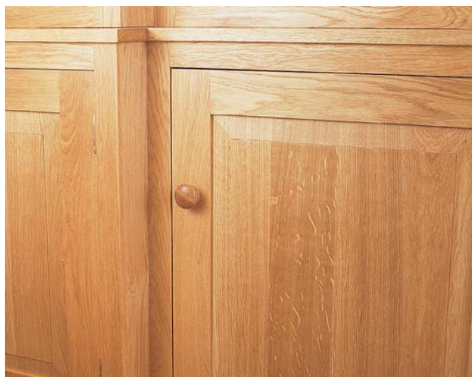
Traditional fielded panels on the doors
