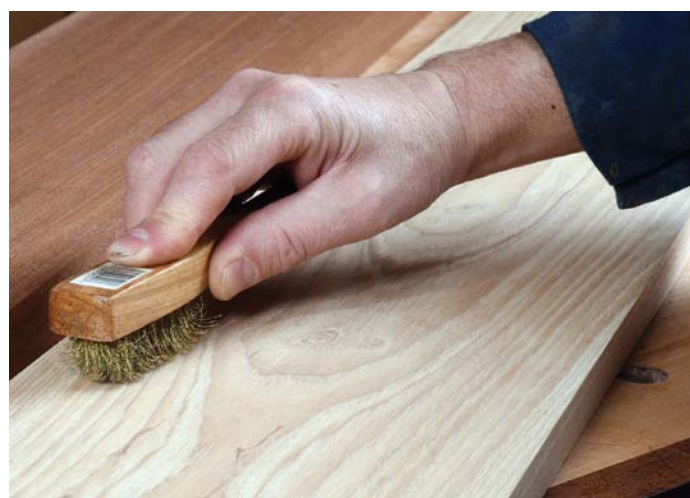
Scrub the grain on coarse timbers for a more dramatic effect
