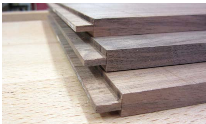
The tenons on the shelf and base cut back to the gauge line
