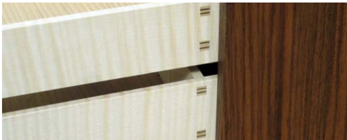
A close-up of the tiny wedged tenons
