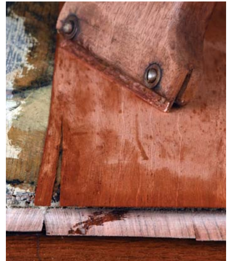
Take care when hammering a dry surface
