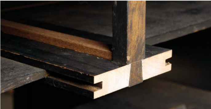
A new hardwood divider was added to the central runner using the original cut nails
