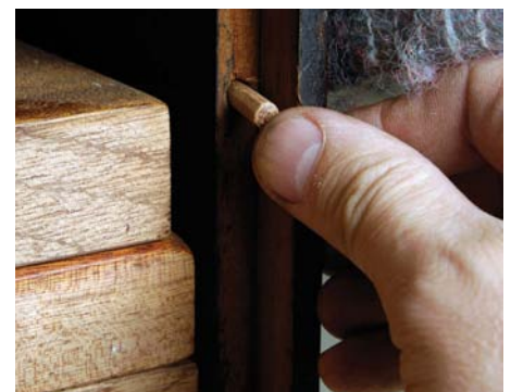
Plug the holes with an appropriate material
