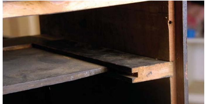
The original runners are returned to the carcass facing up the other way
