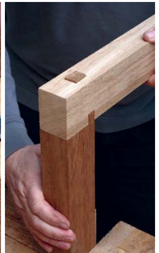
Once engaged the narrow tenon passes through the mortise while the wide collar prevents twisting
