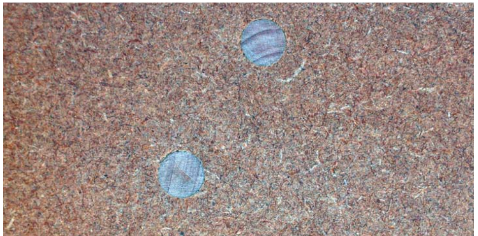
The 'T' section is secured to the base with a number of Miller dowels and the two 'T' elements are similarly dowelled
