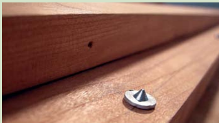
Dowel centres leave small dimples in the bottom of the fence to show where holes should be drilled
