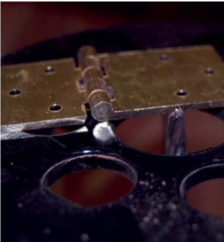
14 I used the actual hinge to set the depth of the router bit before cutting out the recess for the hinge
