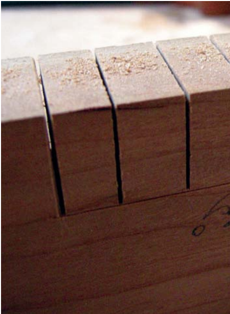
10 A series of cross-cuts within the width of the notch will make chopping the waste much easier
