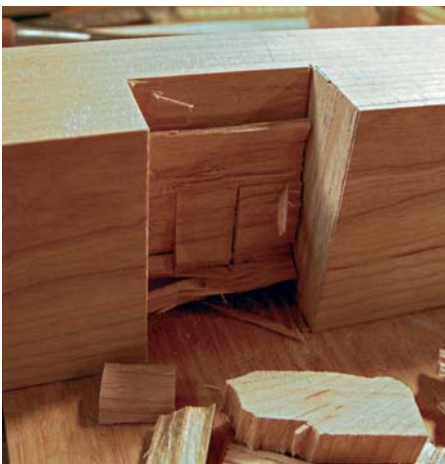
3 Make a series of cross-cuts and remove the waste with a chisel
