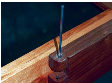
24 Notice the enlarged bore at the top of the knuckle joint to assist pulling out the hinge pin later should the brackets ever need repairs
