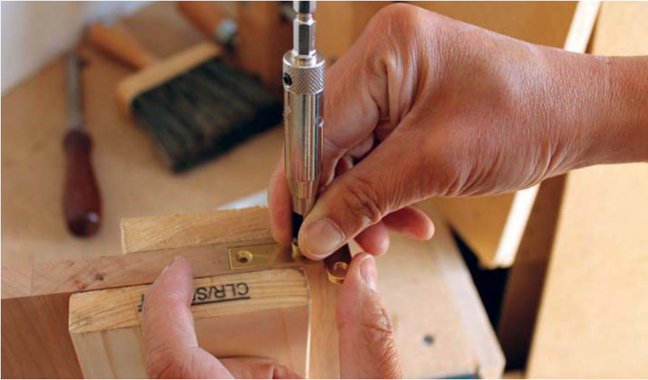
After checking the fit, I predrilled and installed the leaf on the door with screws
