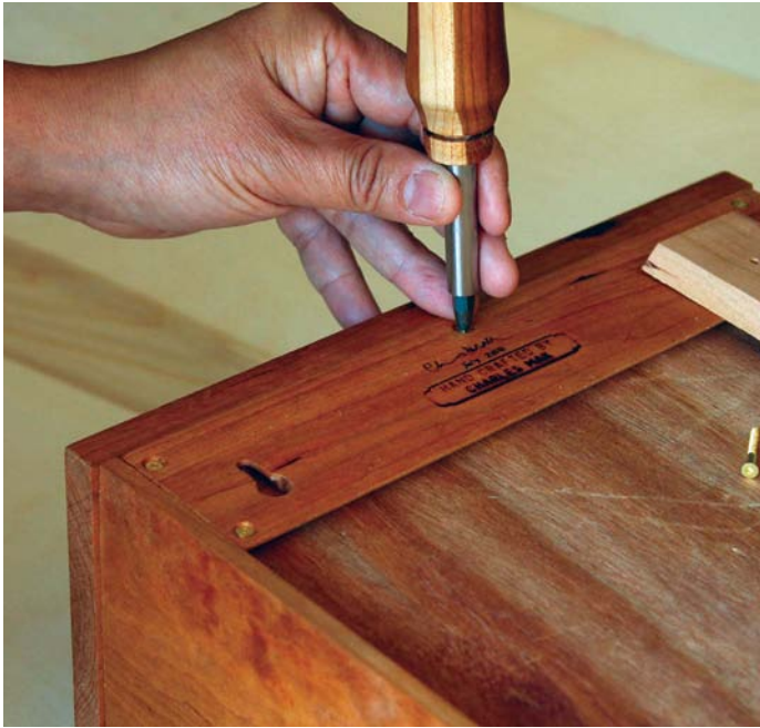
I predrilled and screwed the French cleat to the back
