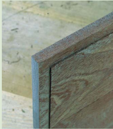
Add a small rebate to the inside of the top and bottom parts
