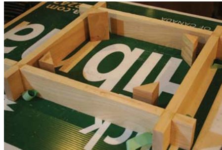
9 The seat frame has a corner block and it is a good idea to glue fix that in place before gluing on the leg
