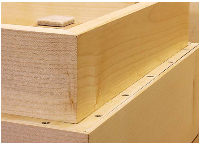
12 The floor is screwed into a rebate in the bottom of the carcass
