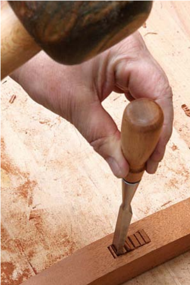
11 A mortise socket is chopped into the post using a vertical chisel for a right angled joint
