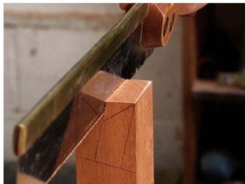
6 The tenon cheeks are hand sawn following the angled lines in the conventional way
