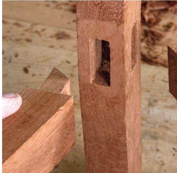
12 Light shines through the L-shaped joint where both mortises meet at the back
