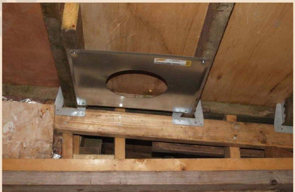
The register plate screwed up to the rafters. This was when I realised that the register plate is designed for a rafter system that runs at 90° to mine. In order to adapt and maintain the clearances to combustible materials I had to make a jury-rigged system
