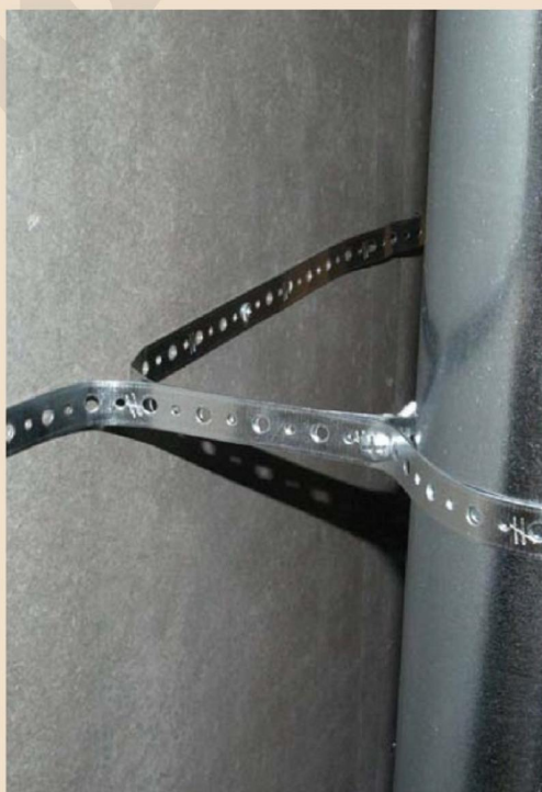
Close up of the flue bracket using fixing band from my local builder's merchant. You can fit as many of these as you like
