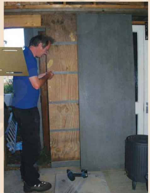
I used a fire-resistant board called Cemboard particleboard behind the flue. The flue gets really hot so it's essential that the recommended clearances are maintained. I'm using strips of Cemboard to make the main board stand off the plywood wall.
