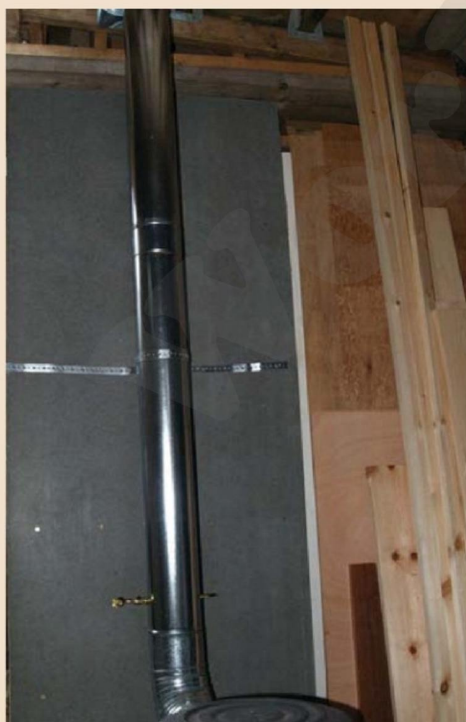
All components loosely positioned and the first home-made flue bracket is fitted
