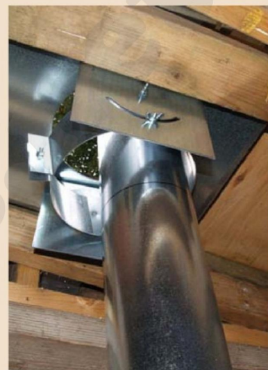
The hole in the roof deck has now been cut
