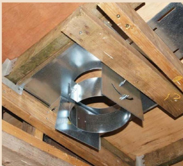
The gimbaled rafter hanger in position. Note I've had to turn it through 90° to accommodate my rafter run. That has required trimmers. At this point I doubled up on trimmers as the rafter bracket provides the main support for the external double skin flue. Once satisfied with the location I replaced the extra trimmer, seen here at an odd angle, with a steel angle beam. This was both extra strong, easy to bolt to and non-combustible
