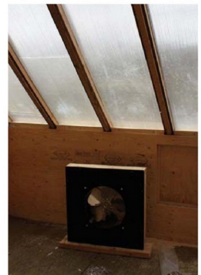
Fans located in the side of the kiln aid airflow through the stack
