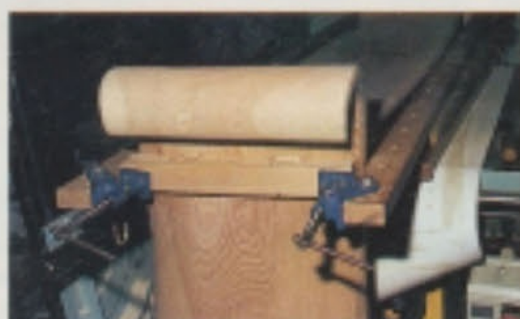
Cramped up – note cut outs on the block for wedges
