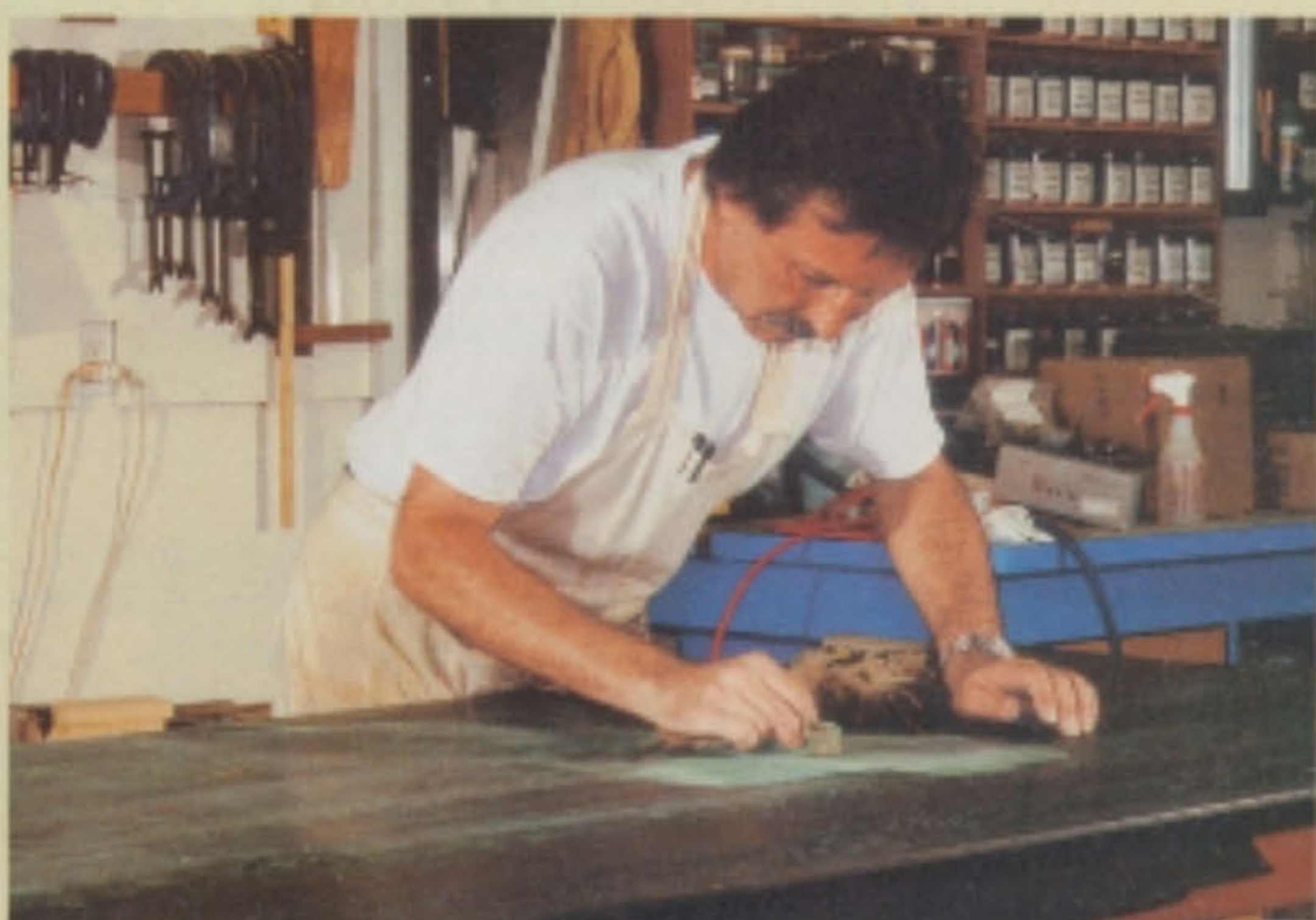
Burnish with hessian across the grain to remove excess plaster
