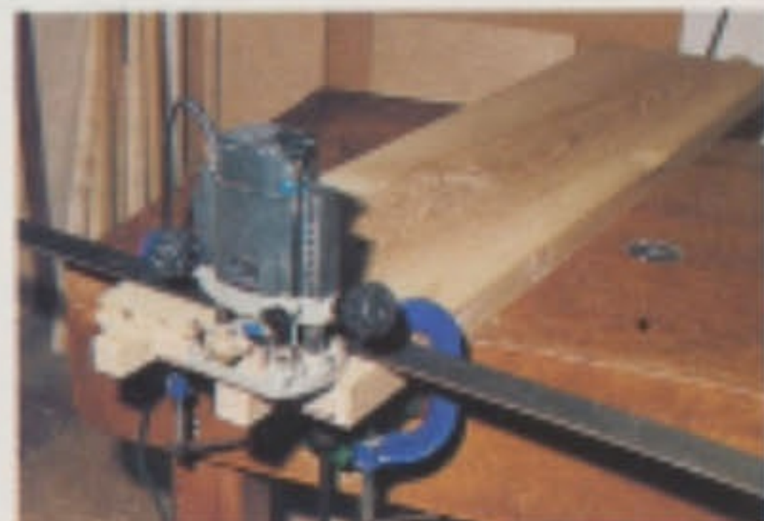
Routing the shoulders
