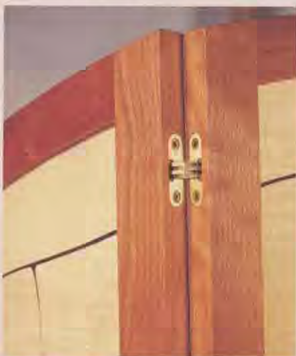
SOSS hinges have a neat appearance and are only seen on the inside edge
