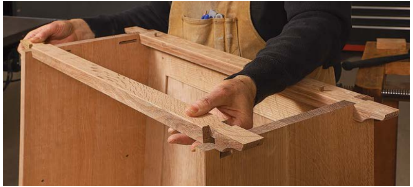
Lockdown. Fit the stretchers into their notches, pressing them down flush with the sides. Then knock home the tusks to lock the sides tight.
