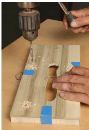
Dowels locate template to frame. Tape the template to the frame, and drill dowel holes in both. Then glue and tap dowels into the frame. The dowels hold the template still during routing, but it's easy to pop the template on and off.
