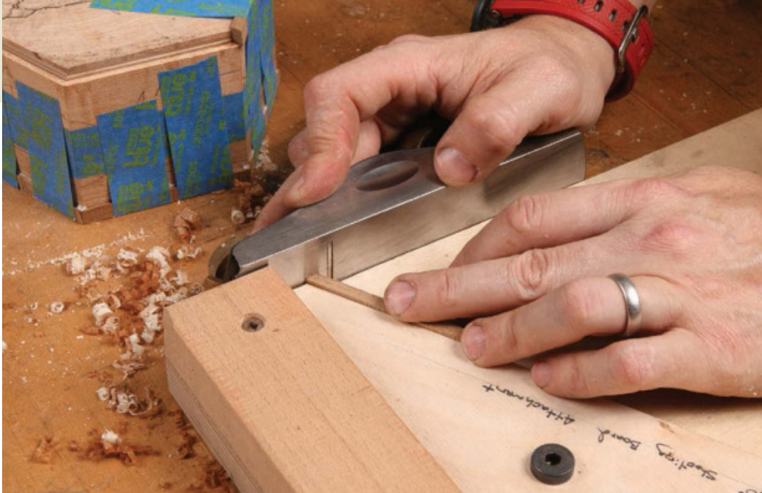
Saw and shoot. Saw the banding to length, and use the 60° bench-hook setup to trim the ends.
