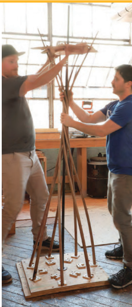
Do the twist. Rotating the upper plate causes all the legs to twist together. The upper plate spins around the metal pipe at the center and is held at the right height by a pin that runs crosswise through holes in the pipe.
