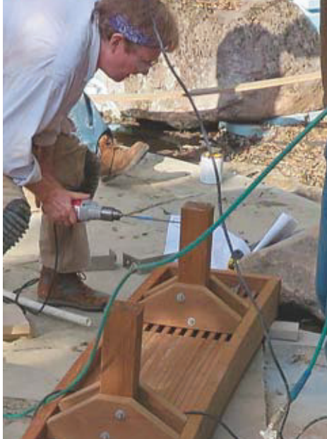
Drilling the legs. Because there might be slight variations in the elevation of the slab, the holes in the legs for the bracket bolts are drilled on site, where accurate measurements can be taken and transferred.
