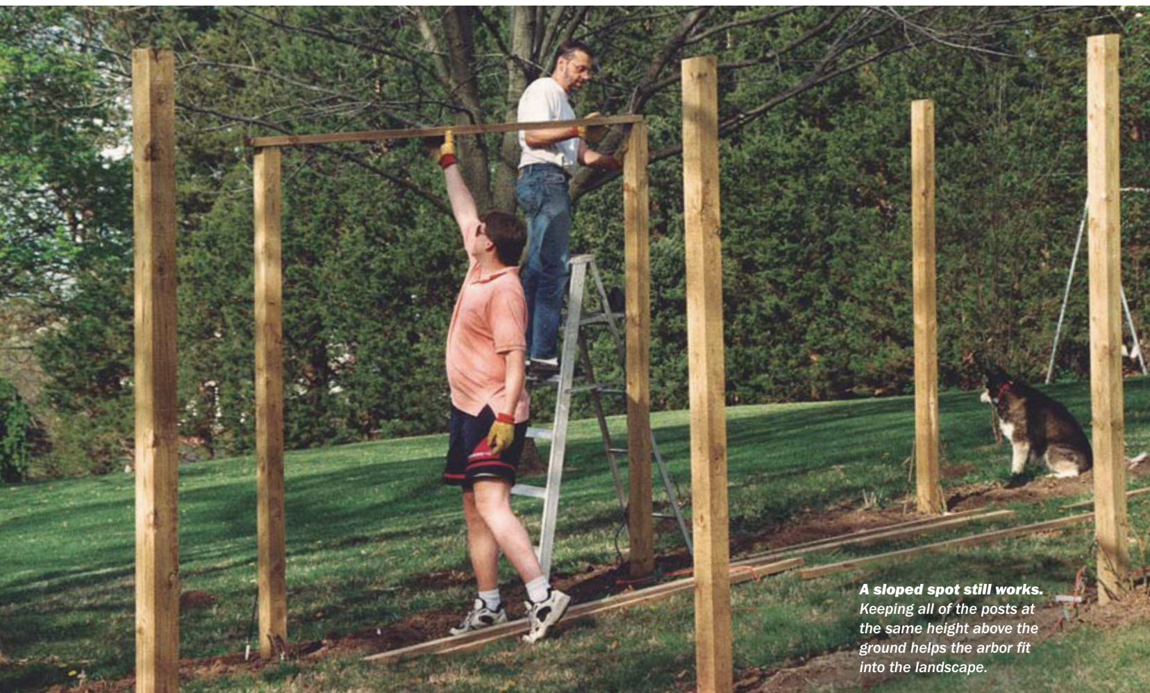
Let a machine do the work for you. With the help of a rented power auger, set the posts in holes 2 ft. deep. A post-hole digger would also get the job done, but more slowly.
