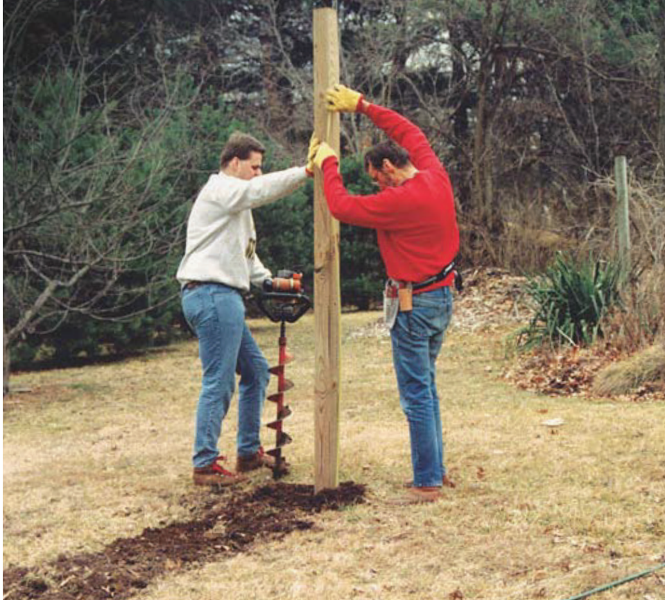
Let a machine do the work for you. With the help of a rented power auger, set the posts in holes 2 ft. deep. A post-hole digger would also get the job done, but more slowly.
