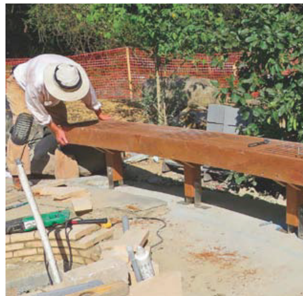
Ready for the masons. With the brackets affixed to the legs, the bench is turned over. The next step is installing the adhesive anchors. Finally, the masons will return and lay the patio stone under the benches.
