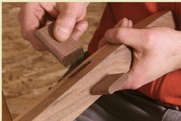
To maximize the length and strength of the slip tenons, Korsak glues them into intersecting mortises, being sure the miters meet. Once the glue cures, he proceeds with the full assembly.
