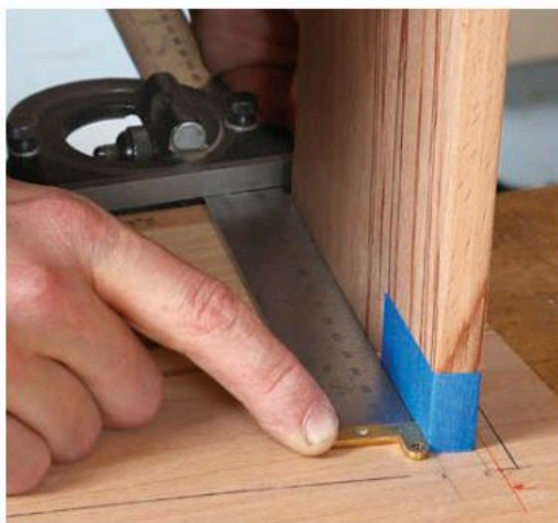
Locate the hinge. Blue tape on the cabinet creates a perfect gap, while a combination square ensures that all the hinges are in the same plane.
