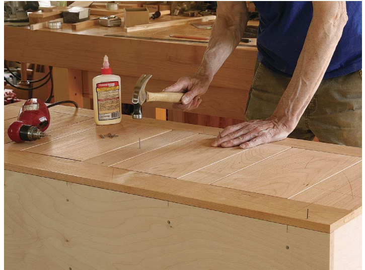
Beautify the back. With the drawer fitting finished, Becksvoort glues the solid cherry frame-and-panel back to the cabinet.
