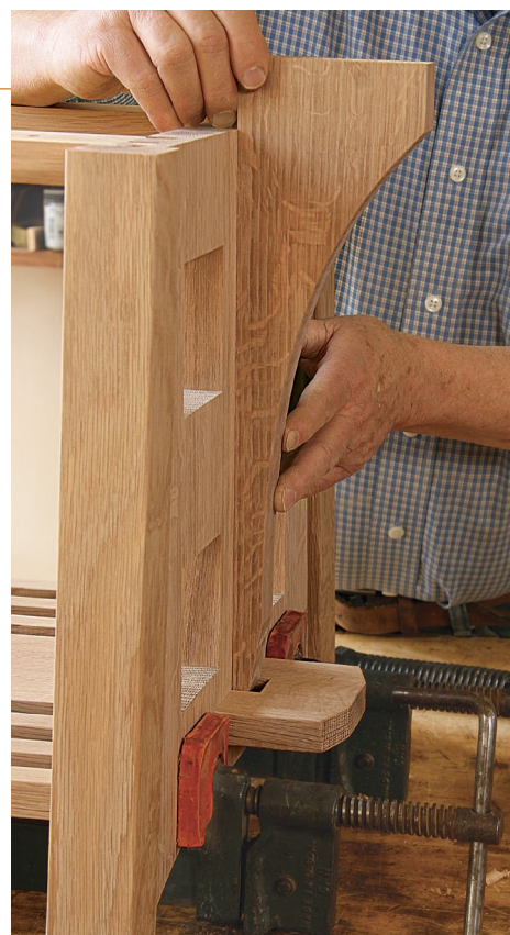
Corbel after clamps. Pull the end panels tight with clamps, then drop the corbel into place.
