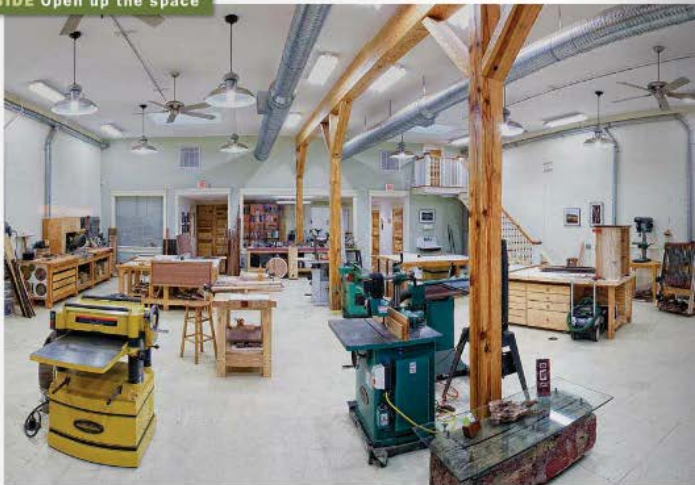
A load-bearing wall in the middle of the space (1) was replaced with 8x8 pine columns topped with a Parallam beam (2). Johnson and Swann encased the beam in heart pine, mitering the corners so it appears solid. Wanting to run dust-collection ductwork and electrical wiring under the floor, they installed a flooring system of 2x6s on edge on top of the concrete slab (3). Then they screwed down two layers of 3/4-in. plywood.
