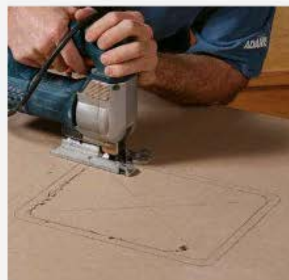
Ready to rout the rabbet. Place the insert plate in the center of the table and trace around it. Then trace another line \frac{1}{2} in. inside the plate outline and cut along it with a jigsaw (above). Now put the plate back in place, and use carpet tape to attach guide strips around it (right).
