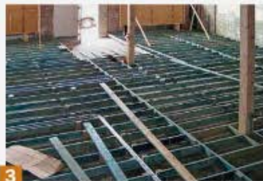
A load-bearing wall in the middle of the space (1) was replaced with 8x8 pine columns topped with a Parallam beam (2). Johnson and Swann encased the beam in heart pine, mitering the corners so it appears solid. Wanting to run dust-collection ductwork and electrical wiring under the floor, they installed a flooring system of 2x6s on edge on top of the concrete slab (3). Then they screwed down two layers of 3/4-in. plywood.
