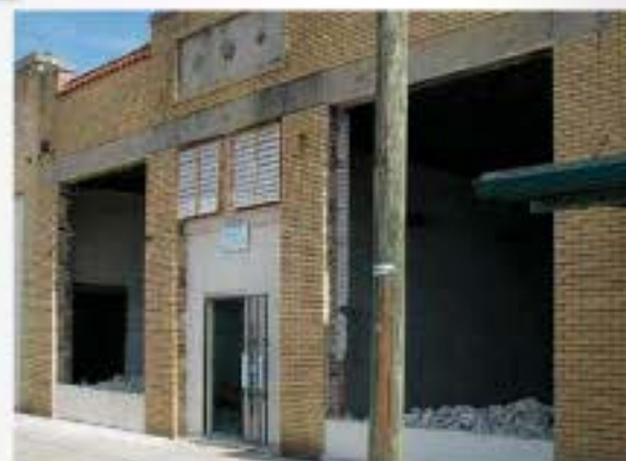
Removing the concrete-block infill and replacing it with glass transformed the space. Once the glass was in, Johnson and Swann installed solar shades made with a mesh fabric that reduces heat gain without blocking the view.
