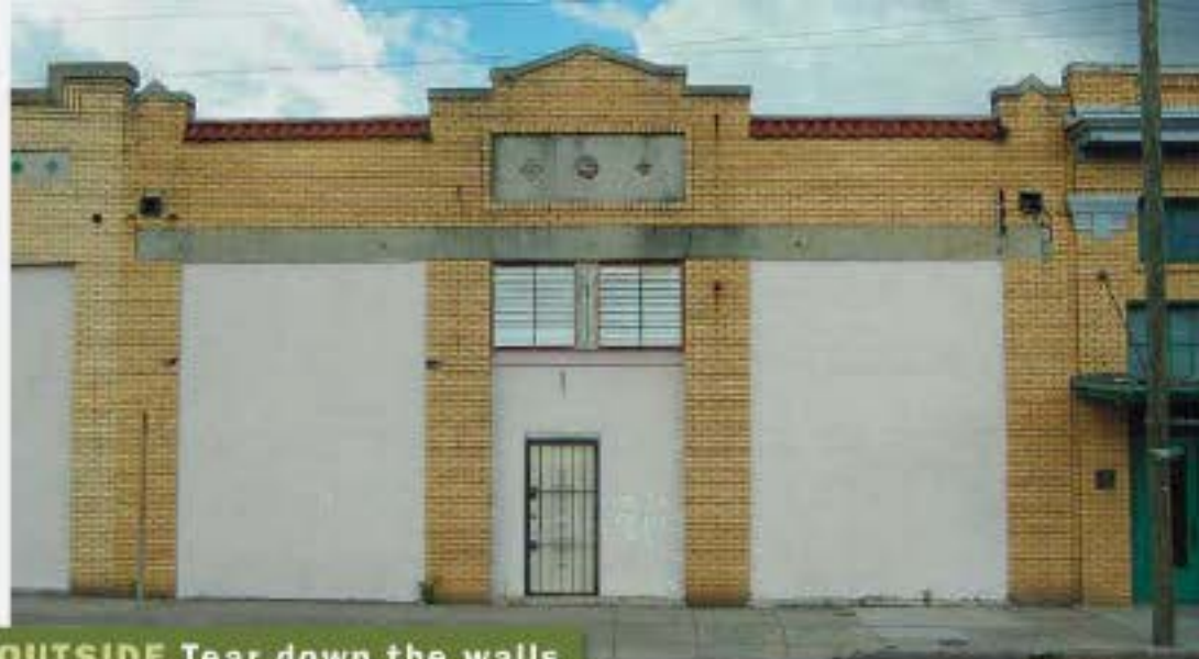
OUTSIDE Tear down the walls
