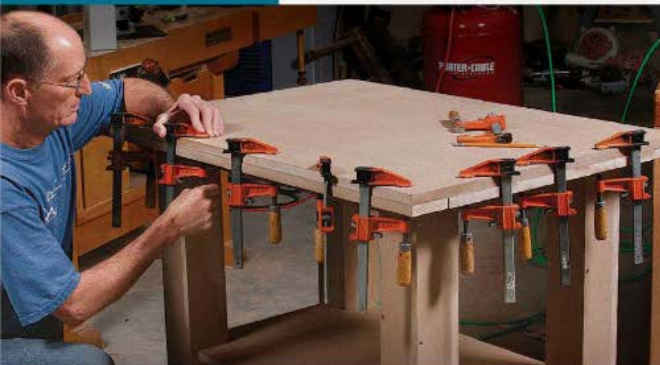
Flip the top and fit the last two strips. Push the first two strips against the base before clamping on the last two, making sure they are touching the base too. If their outside edges don't line up perfectly, just hit them with a flush-trimming router bit afterward.
