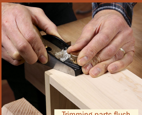
Trimming parts flush
