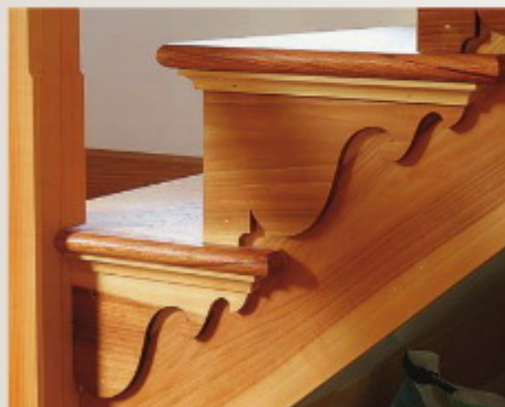
Taking stairs to a new level. The decorative stringer faces, bandsawn to shape, lend a personal touch.
