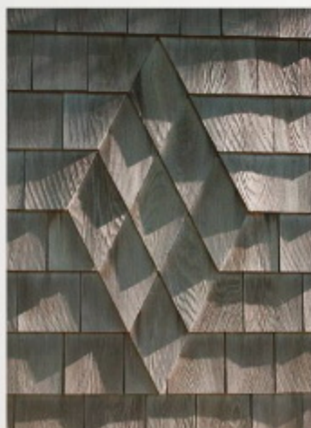
A gem of a detail. Houck cut and installed shaped shingles for decorative touches like this diamond pattern near the shop's main entrance.
