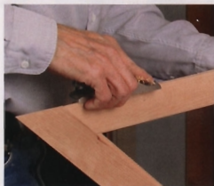
Scribe, fit, and glue it in place. To correct the small gaps on the end cap, Becksvoort runs a compass along the surface of the ceiling (above), transferring the undulations to the frame stock. Then he uses a block plane to shape the frame to that line (left).
