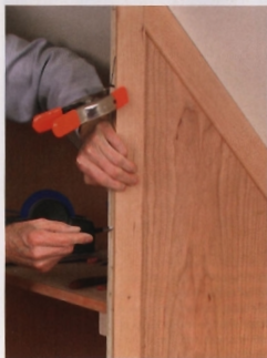
Fit the front edge too. Once the wall side of the frame is profiled, set it in place and use the plywood divider to run a line along the back side of the end cap. Cutting to this line will make sure the front is perfectly flush with the edge of the plywood, which is crucial because the face frame has to land there.
