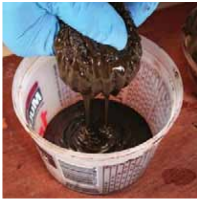
Filter the filler. After adding the colors, squeeze the filler through layers of cheesecloth to mix in the color and remove lumps.
