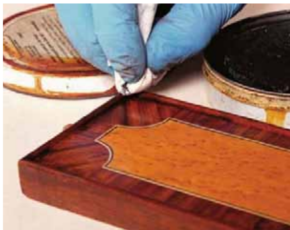
Dark wax in the corners. Wipe on some dark wax, letting it build up in the corners to imitate antiques.
