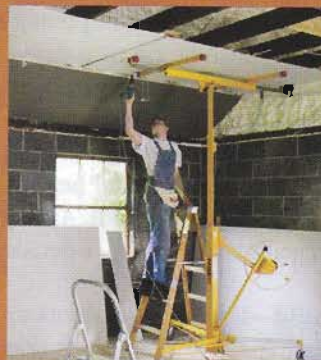
3. Finish the ceiling
