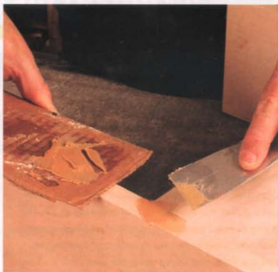
Fill the gap. Use a putty knife to force the filler into the open joint. The color difference will disappear when the filler dries and finish is applied.
