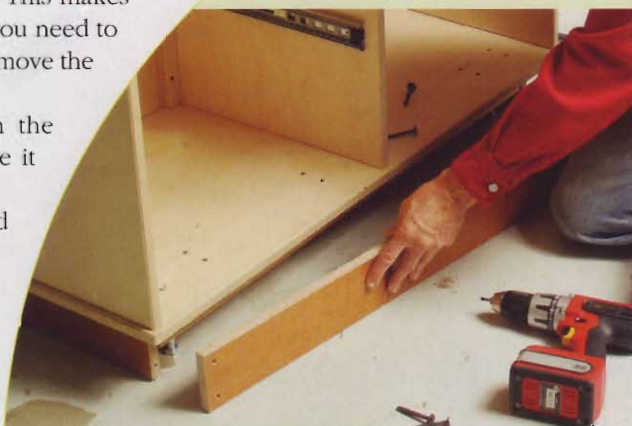
Add a kick plate. The plate hides the feet and stops things from rolling under the cabinet. It's easy to remove to make height adjustments.
