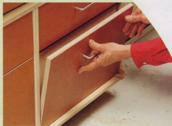
Install the false fronts. Use shims and double-faced tape to position each drawer front, and then screw it on from the inside.
