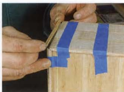
Corners first. Binding strips are glued into the corner rabbets and held with tape. Janofsky uses a Japanese handsaw to separate the sections after the glue has dried.
