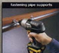
fastening pipe supports
