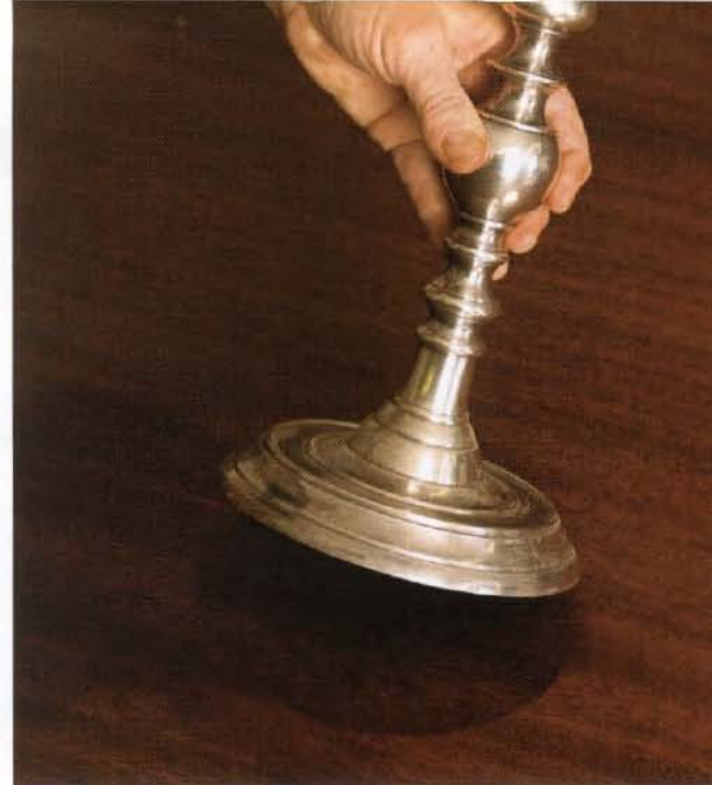
Hidden color. The candlestick protected the tabletop from sun damage, preserving the original darker color.
