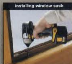
installing window sash
