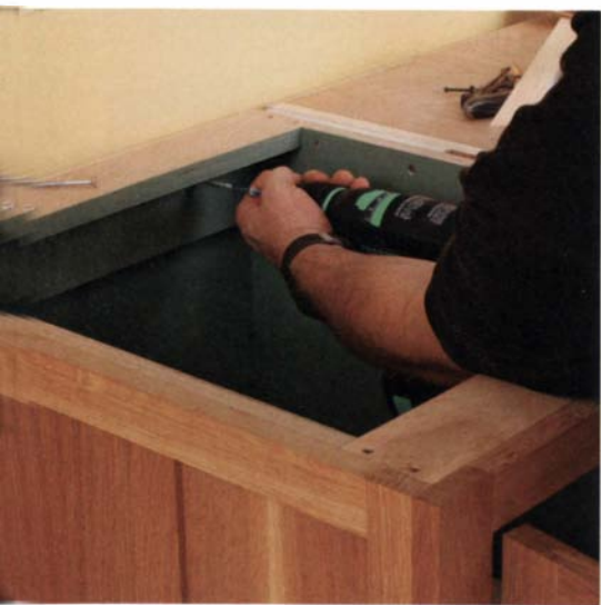
Attach the cabinets to the wall. Drive 3 1/2-in. screws through the cleat and into wall studs to lock the cabinet to the wall.
