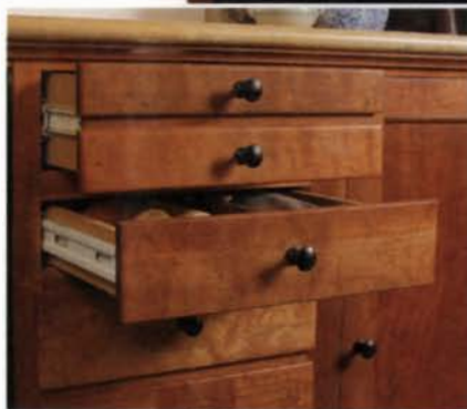
Graduated drawer fronts. To mimic the Shaker style, the author designed the drawer fronts so they get narrower near the top. Note that the top two faces are really one drawer, built to a more useful size for a modern kitchen.
