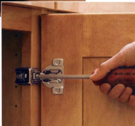
An open-and-shut case. Euro hinges lend a clean look to a cabinet's exterior (top) but can't do the same for the inside. What they lack in looks, they make up for in adjustability.
