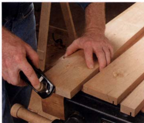
Prepare the face-frame pieces for installation. Chamfered edges hide inconsistencies at the joints, allowing you to prefinish the parts in the shop and nail them on one at a time.
