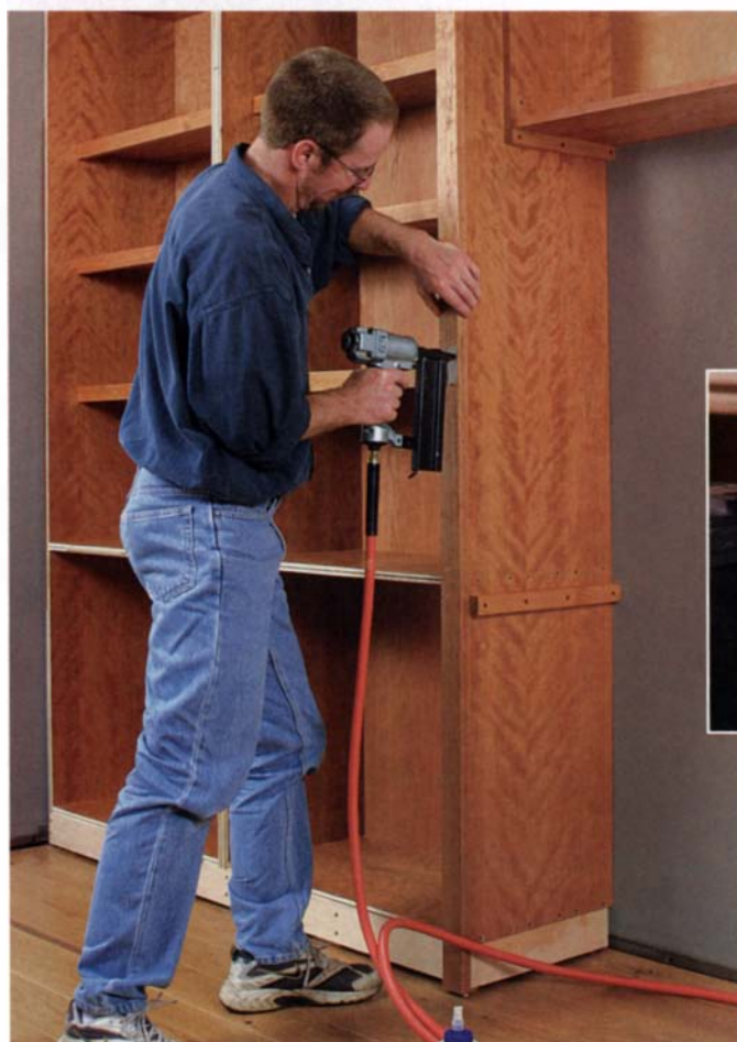
Start with the innermost stile. This joint must be flush. Adjust the alignment as you nail on the piece. Shoot through a thin piece of cardboard if your gun has a tendency to dent the surface (inset). Later, fill the nail holes with colored wax.
