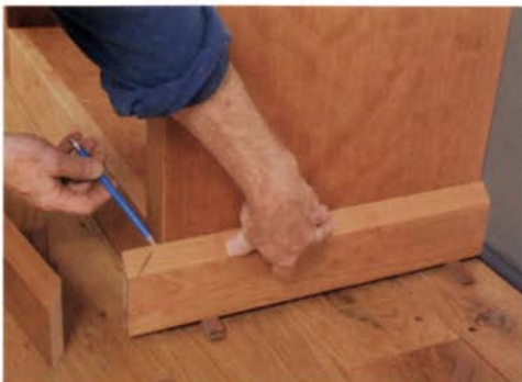
Install the base molding. Starting with the return piece, shim the molding up to its proper height and mark the miter (above). Cut the return, and mark and cut the front piece, then nail the moldings in place. A small shoe molding will hide the gap below (see the drawing at left).
