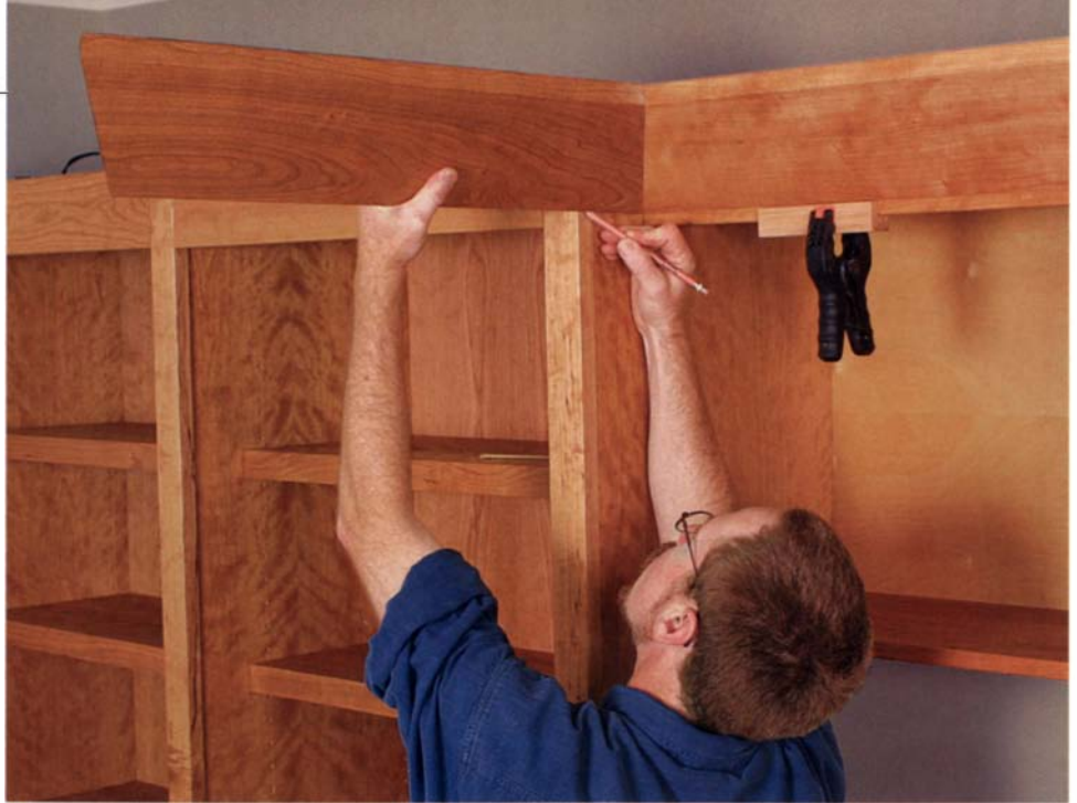
Work from the center out. Clamp blocks to the face frame to ensure an even reveal. On the return pieces, fit the miters first, then dry-fit the pieces and mark their lengths. The front pieces will be trickier. You must nibble away at each end to creep up on a good fit.
