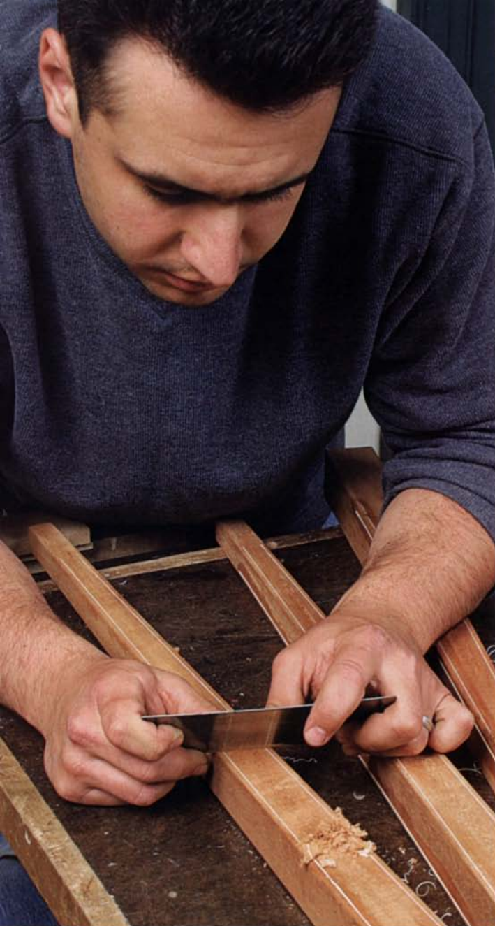
Last, scrape the surface flush. Scrape just enough to clean the surface but not enough to cut beneath the shallow stringing.
