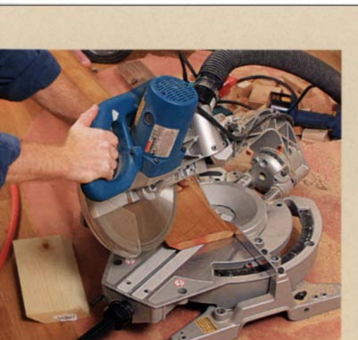
Make test cuts to fine-tune the fit. You will have to reverse the saw fence to cut the opposite angle.
