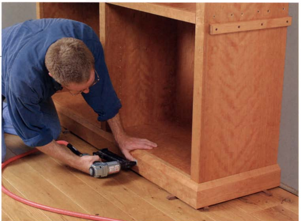
Install the base molding. Starting with the return piece, shim the molding up to its proper height and mark the miter (above). Cut the return, and mark and cut the front piece, then nail the moldings in place. A small shoe molding will hide the gap below (see the drawing at left).
