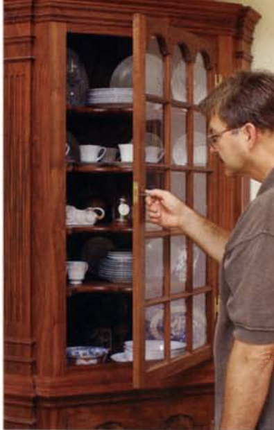
The lockset installed on this door is typical of those found on most 18th-century doors and drawers. It is mortised into the back of the door. A mortise in the opposing door or case captures the bolt.
