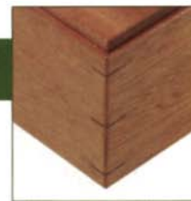
Tenderized veneer. If the veneer spline is too thick to slide into the sawkerf, a few hammer blows will persuade it to fit.
