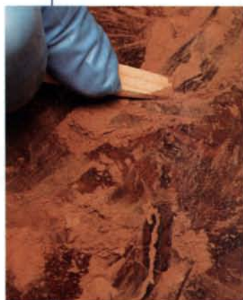
Pack, fill, spray. Fill the gap with sawdust using a wedge of wood to pack it down (left). Add several drops of cyanoacrylate glue (middle), then spray accelerant on top of that (right). The accelerant hardens the glue instantly, making it ready to be worked.
