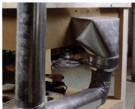
An inexpensive connection. Brown used a standard sheet-metal air-conditioning duct to tie the sanding table to his shop dust system.
