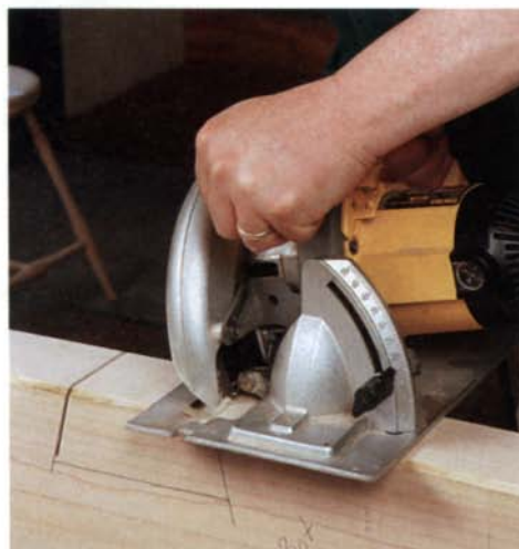
Circular saw comes in handy again. Cut the shoulders first, then cut some kerfs through the waste section.
