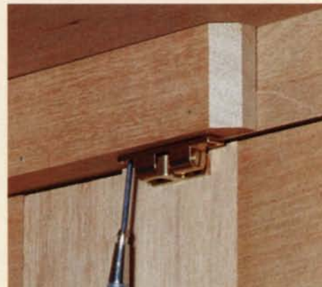
Double-ball catches can be used with lipped or unlipped doors. The female part, shown with the male half engaged, is screwed to a block inside the top of the case.
