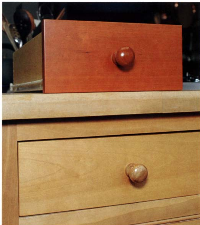
Way too much sun. The cherry kitchen cabinet at the bottom has been bleached from 12 years of direct sunlight through a window facing south. The drawer on top is from another cabinet facing north. The ambient indirect light has given it the deep red patina usually found on the surface of cherry.
