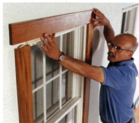
A strong and simple joint. Biscuits not only align the casing header to the left and right members, but they also offer plenty of strength to the basic butt joint.
