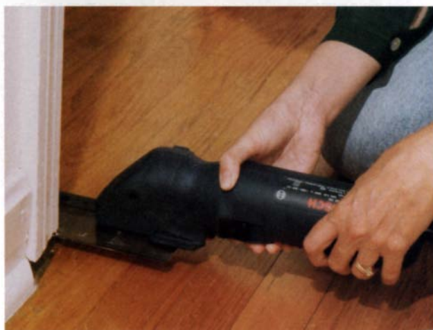
A saw for tight quarters. Bosch's fine-cut saw makes quick work of trimming the bottoms of door casings to fit a new floor or rug.
