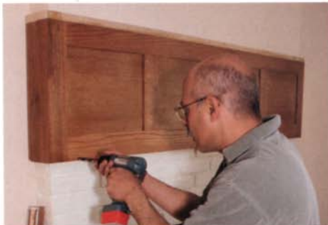
Overmantel slides onto the wall. With the overmantel shimmed level, driving a few screws ties it to the wall.
