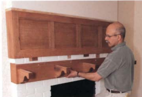
Skirt abuts the overmantel. Shims guarantee that the overmantel and skirt meet flush.
