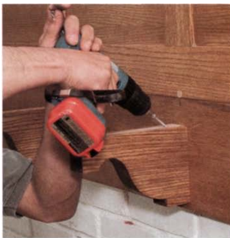
A screw locks the bracket. After the skirt is tied to the wall, a screw is driven at 45° to hold the bracket permanently in place.
