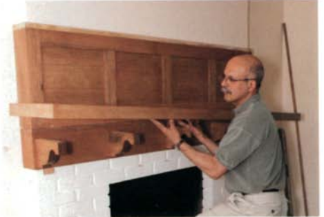
Shelf fits easily onto the brackets. Using reliable measurements in the planning stage ensures the shelf seats itself perfectly level.
