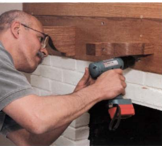
The brackets twist away. When the skirt slides over the brick, the lag bolts allow the author to twist the brackets for easy access to a hidden spot to sink a screw.
