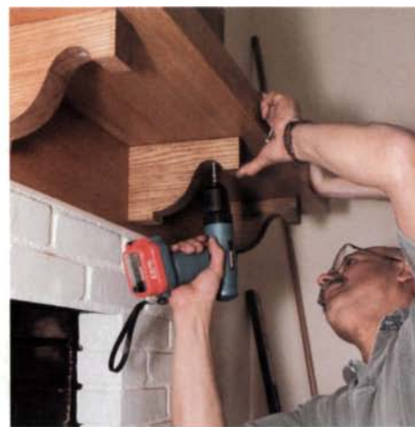
Shelf is attached from underneath. The shelf goes onto the brackets, and an inconspicuously placed screw keeps it there.
